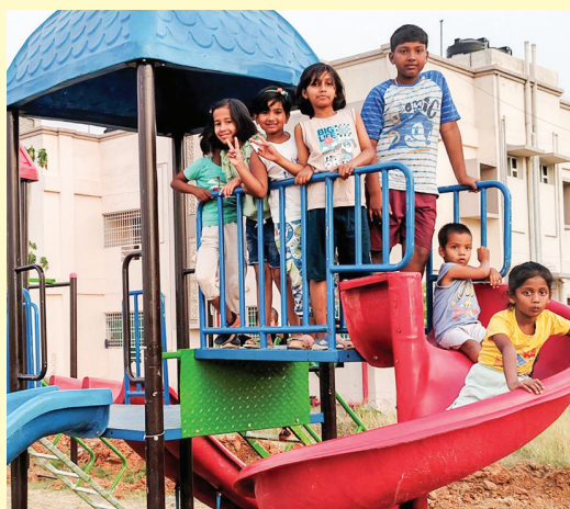
Fig 24. Installation of Multi-Play Children's Park
